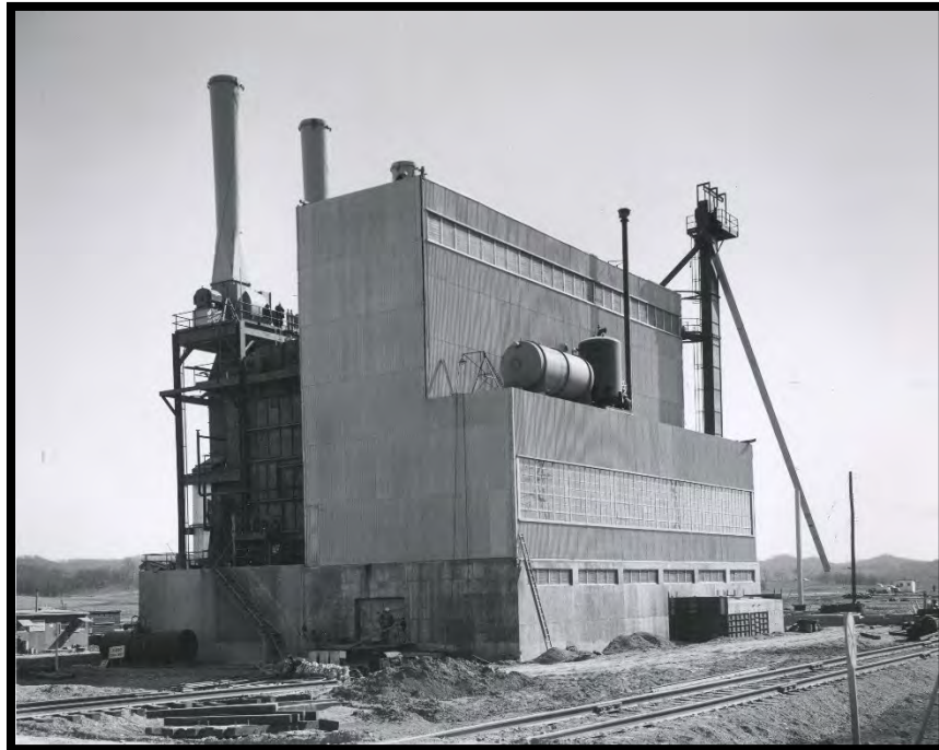
Figure 16: The X-600 Steam Plant, January 1954
