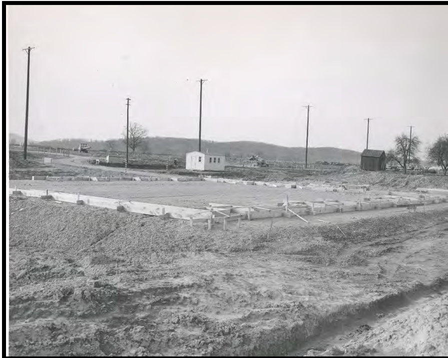
Figure 8: Grading and Foundation Work for the X-600 Steam Plant, July 1953
