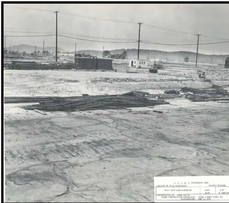
Figure 5: Grading and Foundation Work for the X-600 Steam Plant, June 1953
