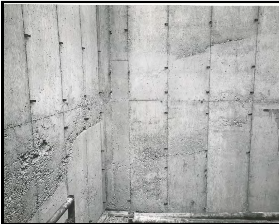
Figure 9: Foundation Work for the X-600 Steam Plant, July 1953
