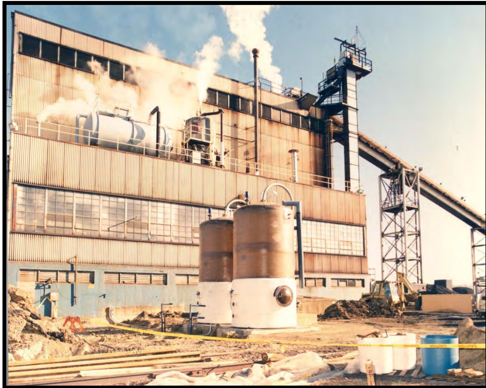
Figure 20: The X-600 Steam Plant, 1990
