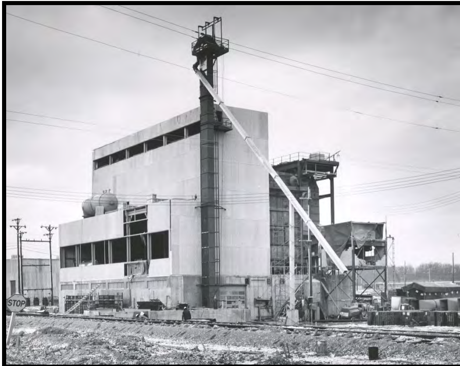
Figure 14: The X-600 Steam Plant, December 1953
