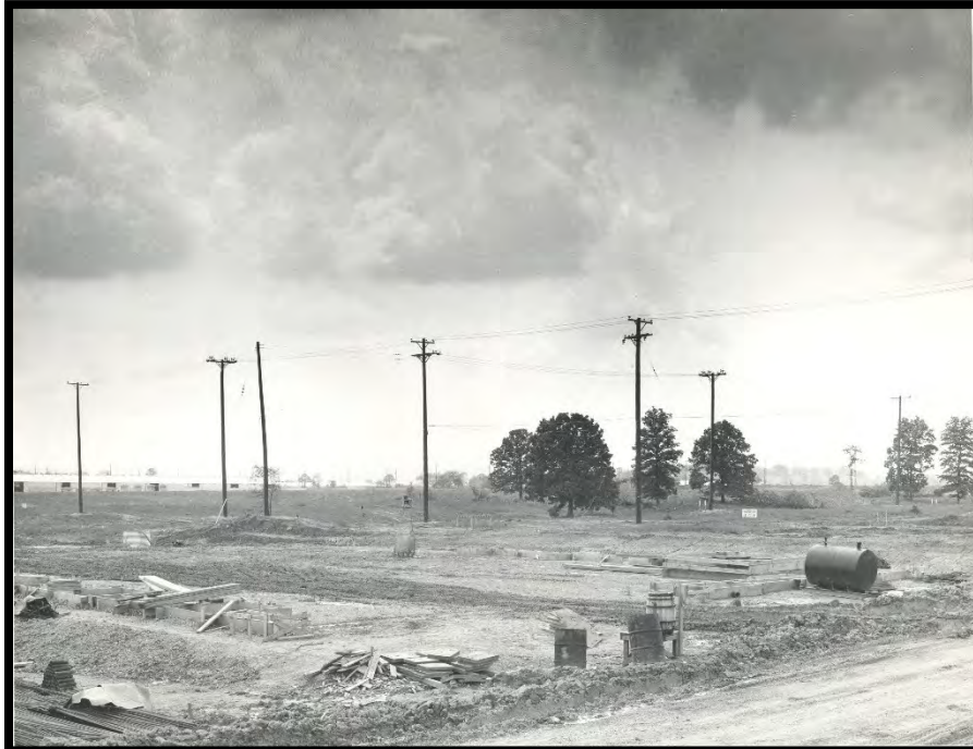
Figure 4: Grading Work for the X-600 Steam Plant, June 1953
