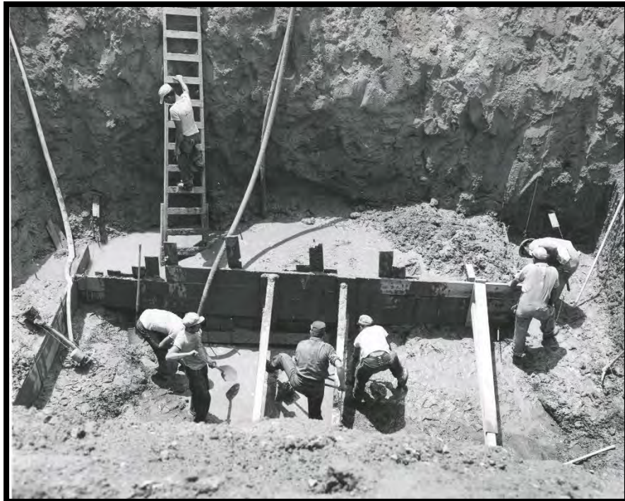
Figure 6: Excavation Work for the X-600 Steam Plant, June 1953
