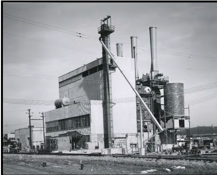
Figure 15: The X-600 Steam Plant, December 1953
