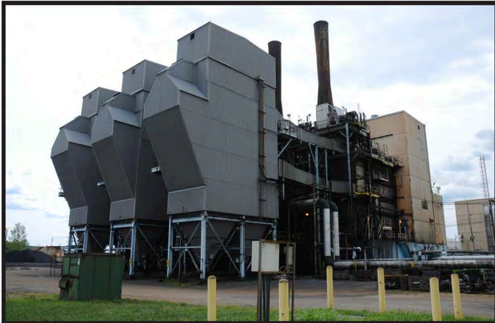
Figure 3: North Side of the X-600 Steam Plant, August 2012, Facing South
