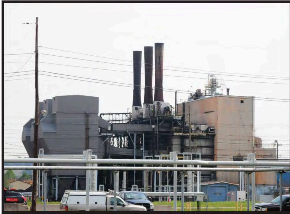
Figure 2: North Side of the X-600 Steam Plant, August 2012, Facing South
