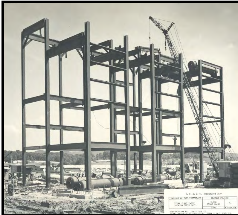
Figure 10: Steel Framework for the X-600 Steam Plant, Looking South, August 1953
